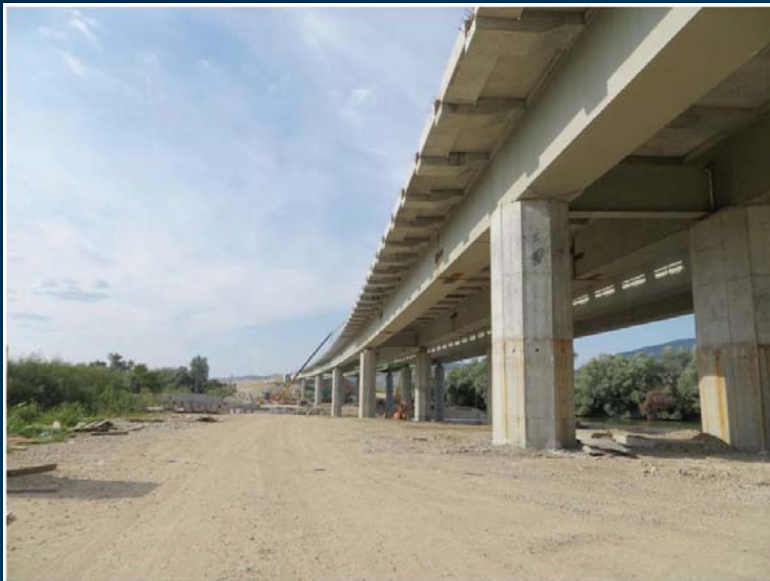
View of the final bridge
