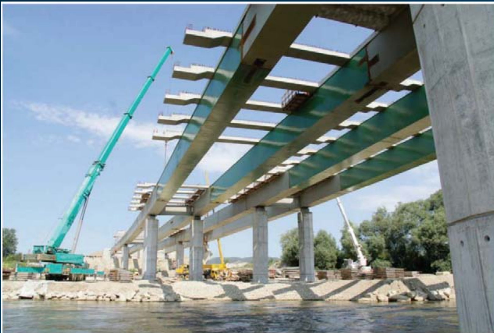
Arrangement of the prefabricated cross girders at equal intervals on the steel boxes
