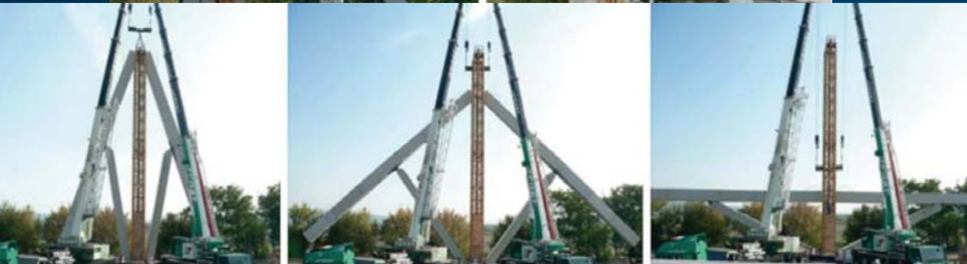
Lowering of the top points of bridge girders with the aid of mobile cranes
