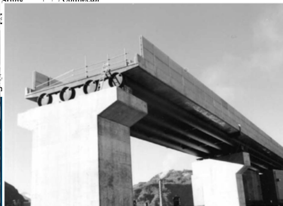
Completed pipe girder bridge.
