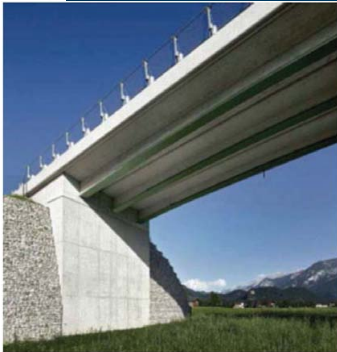
Bottom view on the VFT-WIB girders at Kuchl bridge (A)
