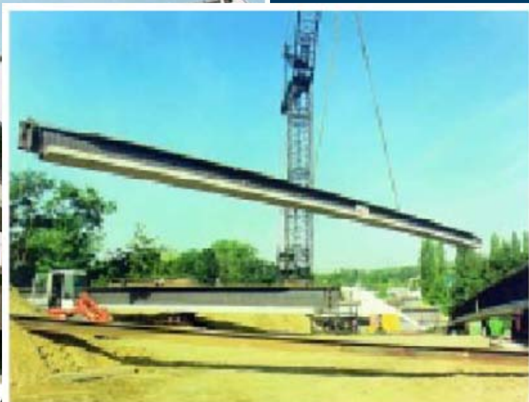
Single span bridge in Kerpen Horrem, Germany. 41,25 m long HE 1000 A beams used for prestressed composite girders of "Preflex" type.
