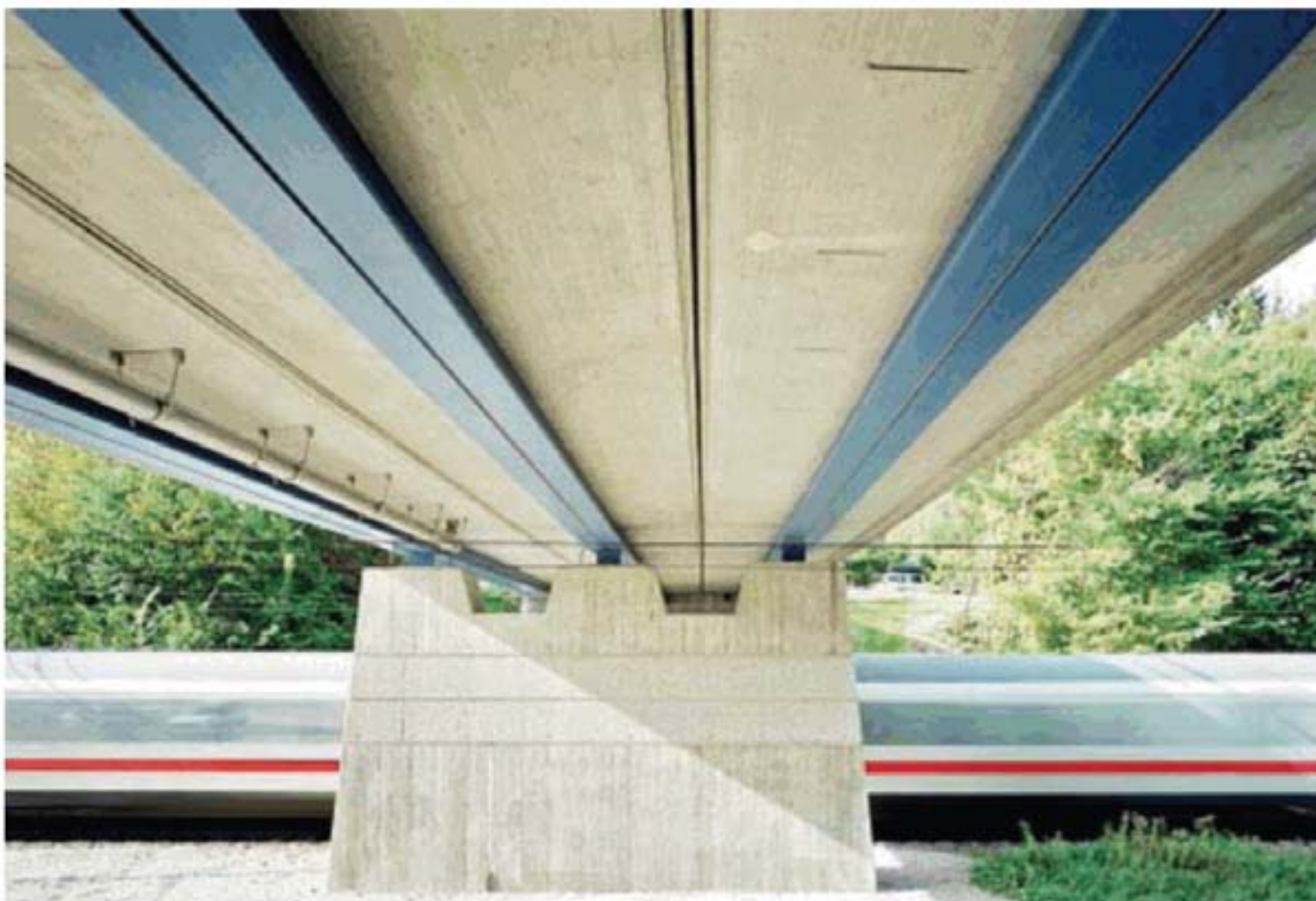
Bottom view with three VFT-WIB girders and spring plates at the middle support
