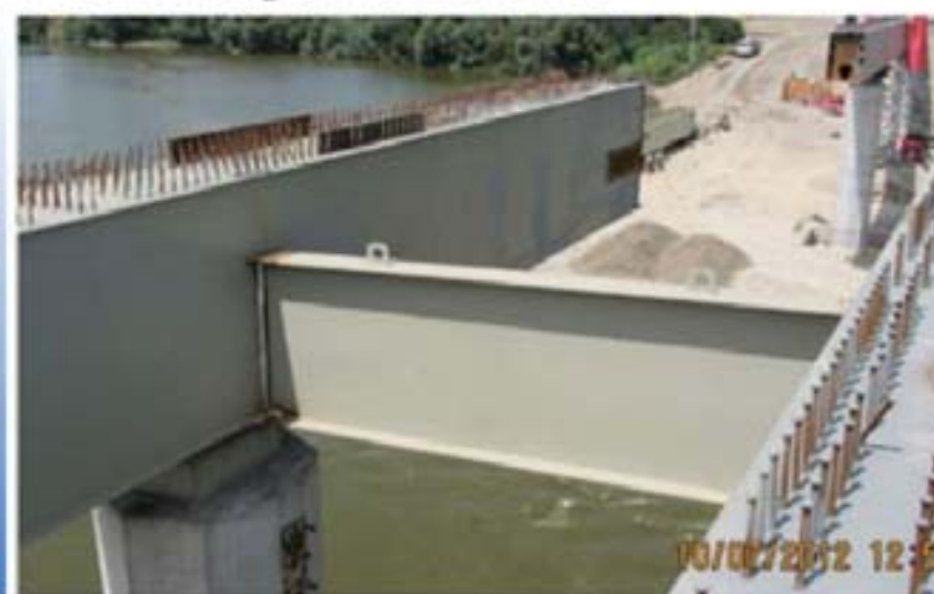
Node with calotte bearings, axes 0 – 4, 8 – 12 – double composite structure
