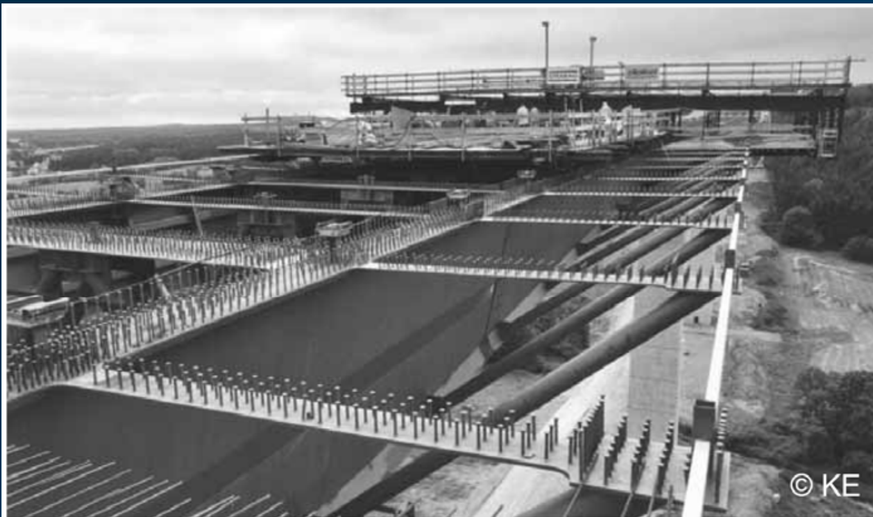
Small stands as support for formwork carriages “running on top”, valley bridge Reichenbach near Ilmenau, Germany, 2002.
