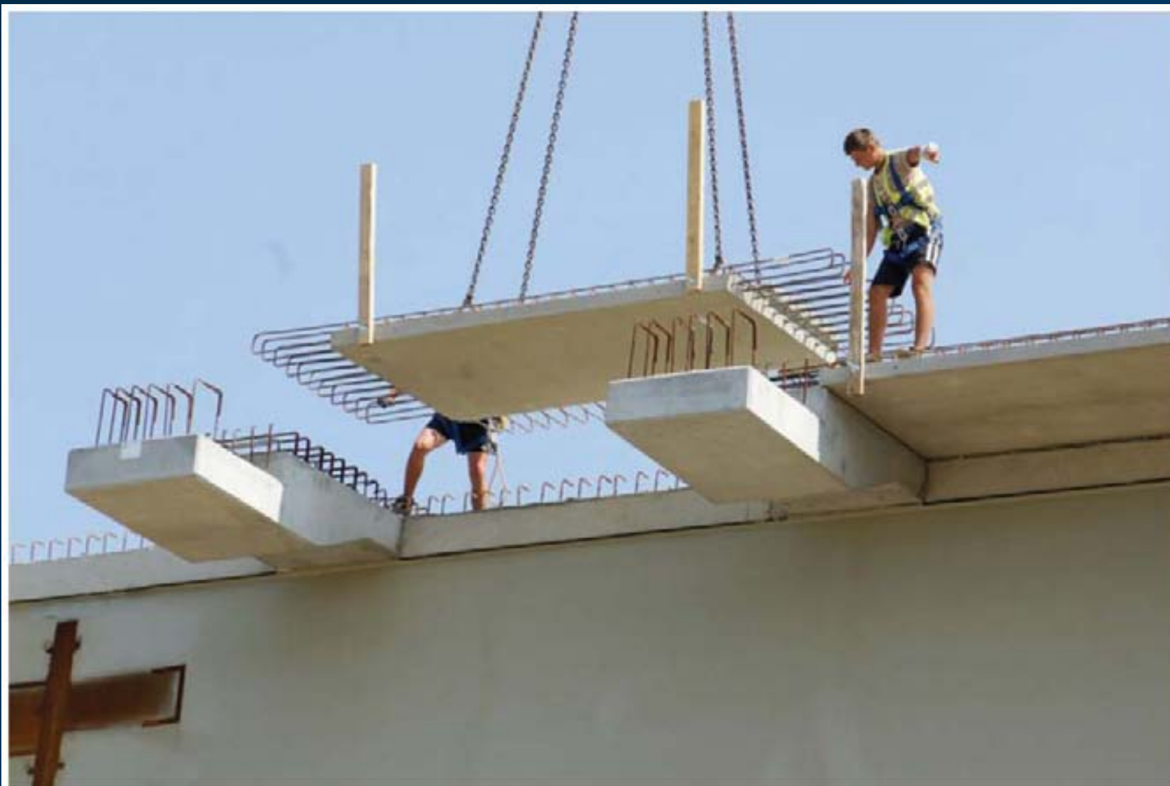
Arrangement of the prefabricated slabs on top of the composite girder system
