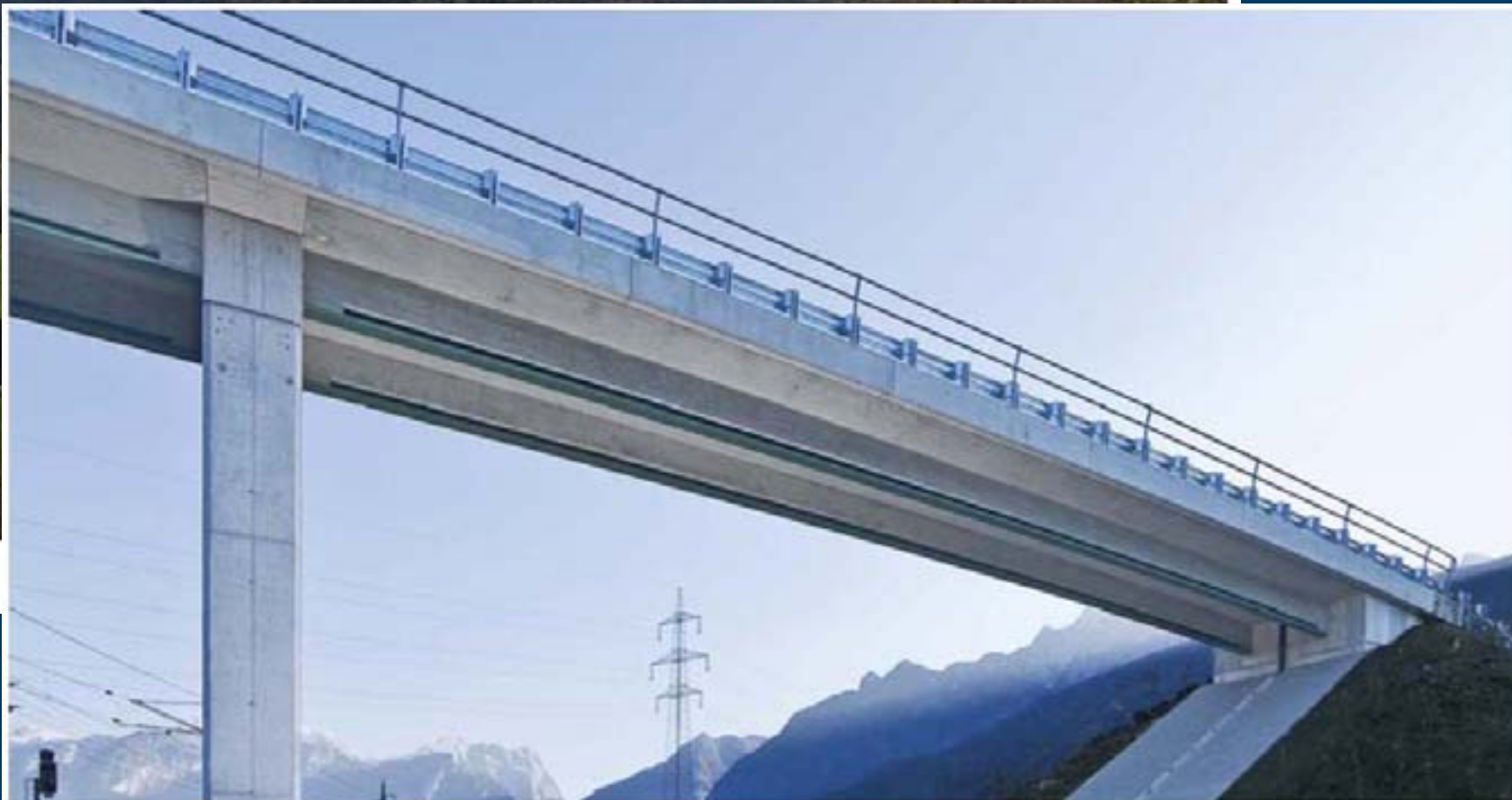
Bottom view of Vigaun bridge
