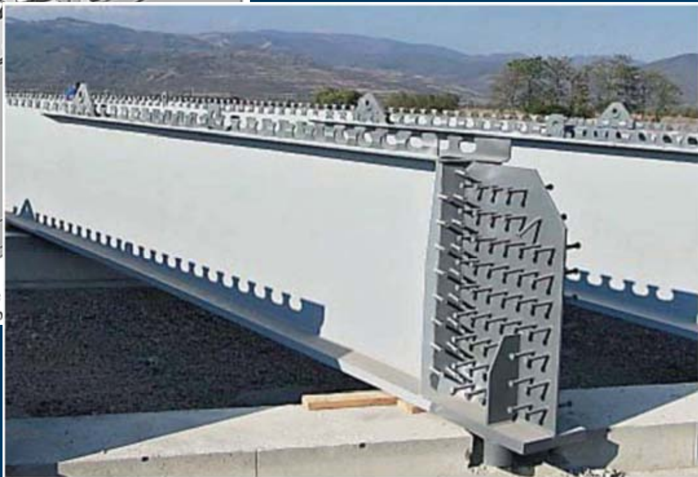
Steel girders on site
