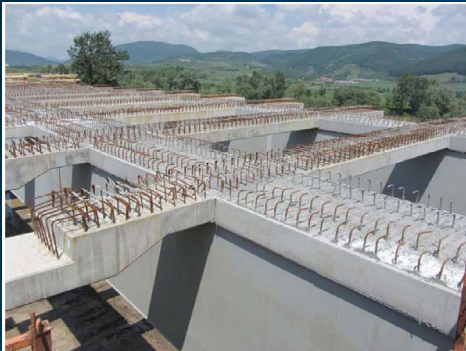
Intermediary composite girder system
