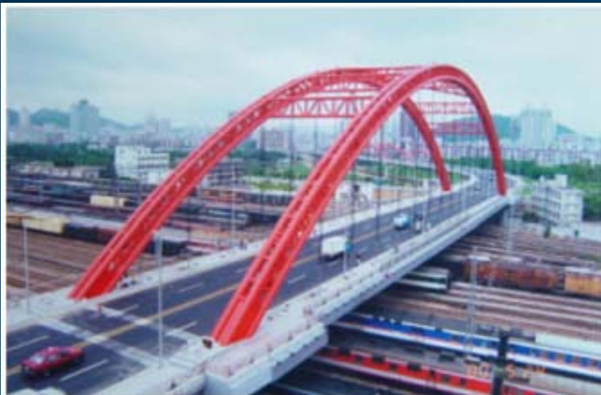
Shenzhen Beizhan Bridge
