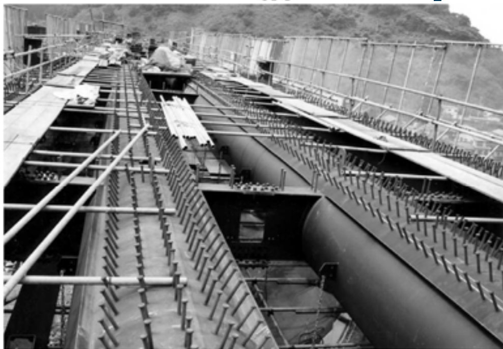
Upper side of the under construction pipe girder.
