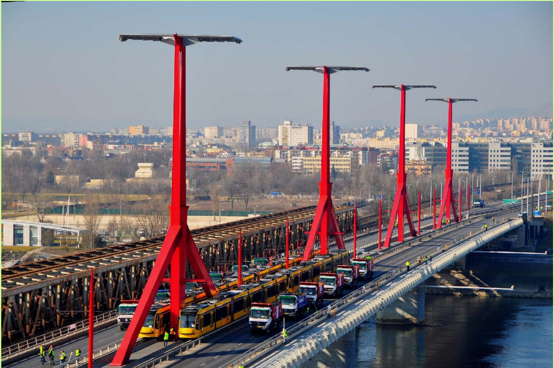
The realized structure (Photo by Tamás Simonyi at the load testing of tram track on 15 February 2015.)
