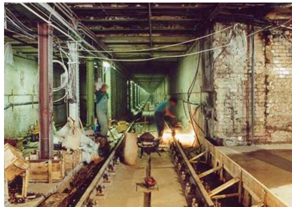
The new track is under construction
