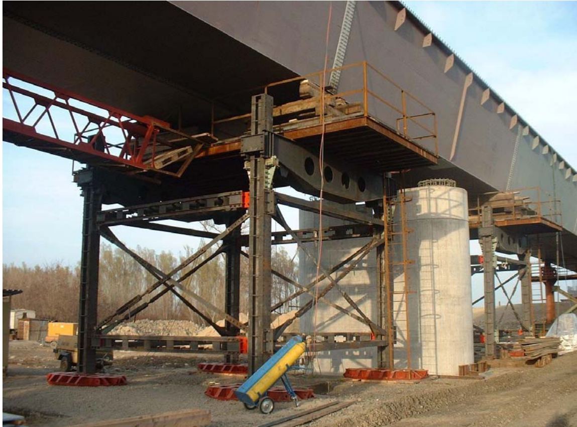
Temporary support made of REM 500 type structure
